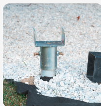
SET LEVEL AT GRADE
